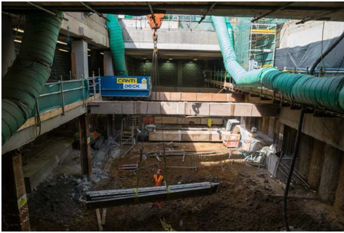
Victoria station north ticketing hall lifting operations
