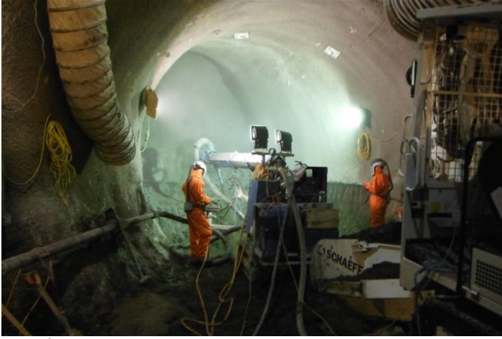
Bond Street station shaft | excavation works
