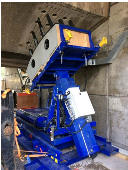
Installation of a concrete anchor block onto the flyover
