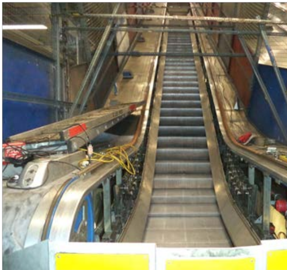
Canada Water escalator installation
