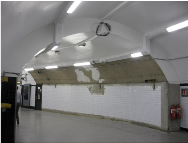
Completion of mid-concourse floor and wall tiling at Chancery Lane
